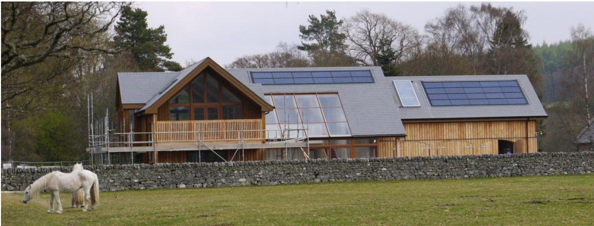
Figure 7.2: A New Build Dwelling in the CNP with Solar PV and Solar Thermal Panels (Source: SAC)
