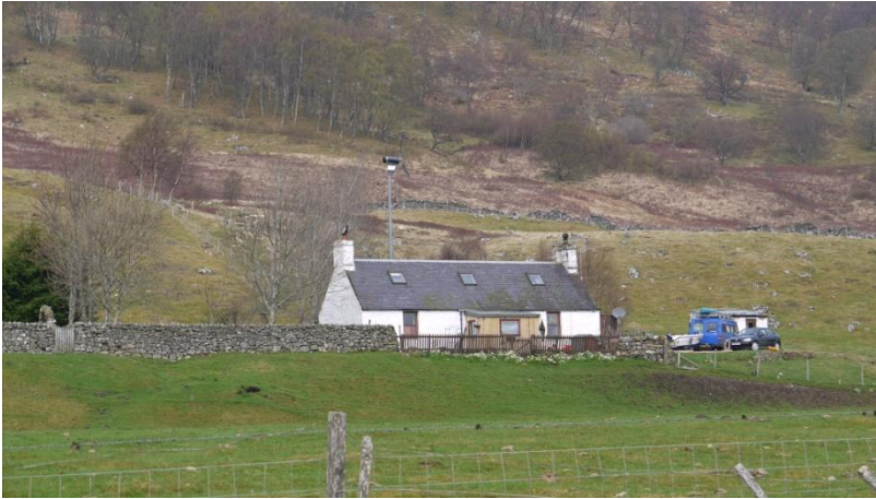
Figure 4.1: Micro Scale Wind Turbine in Laggan Area of the Park (Source: SAC)
