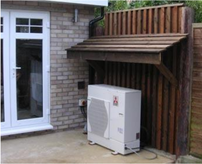
Figure 8.1: Example of a Domestic ASHP (Source: GrEnergy)
