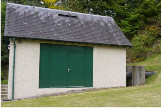
Figure 5.1: A Turbine House for a 940 kW Turbine in Rural Perthshire (Source: SAC)
